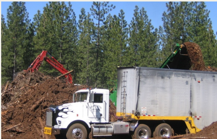
Grind and Haul Biomass Waste
